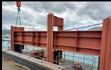
Pile Stress Compound Beam
